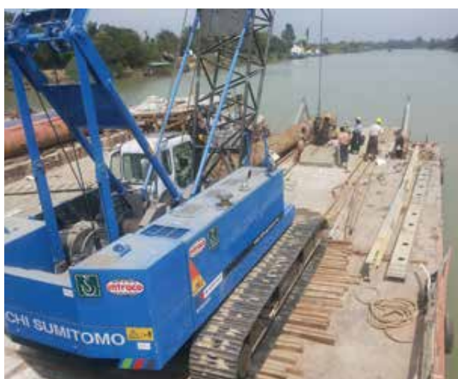
A 55-tonne crawler crane on a bridge construction project in Myanmar.
